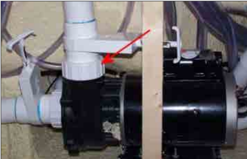
FIGURE 1.2 : PUMP UNION; LOOSEN UP TO BLEED AIR
